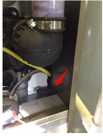
Junction box supplied with unit not installed in furnace to protect 120 volt electric splices. Top of furnace case bent downward at middle, making installation of sealed cover difficult. Recommend review by a licensed heating contractor
