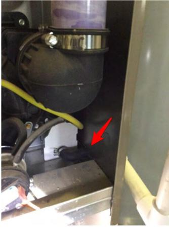
8: - Junction box supplied with unit not installed in furnace to protect 120 volt electric splices. Top of furnace case bent downward at middle, making installation of sealed cover difficult. Recommend review by a licensed heating contractor
