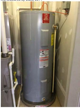
Electric water heater. Shut off valve present for cold water to unit. A Temperature Pressure Relief (TPR) valve is installed as a safety feature
